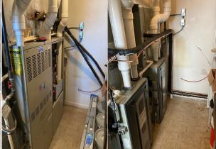
**First Federal Savings and Loan, Swanton** – GEM Service techs replaced two split systems, furnaces, air conditioners and a hot water heater.
