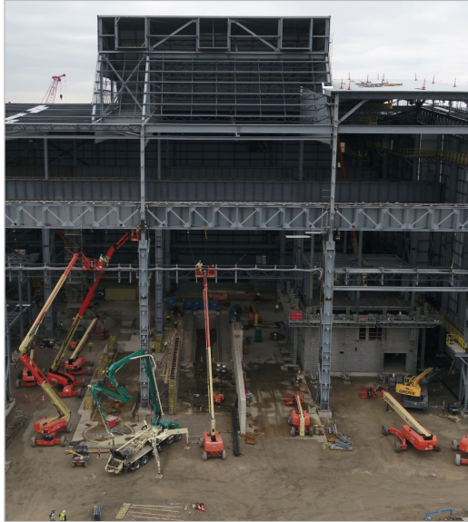
Left: North Star melt shop - masonry walls going up, foundations being poured and lifts for finishing steel.
