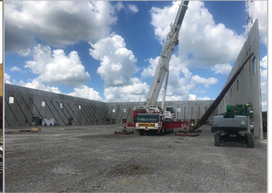
At left, RLI cement finishers place concrete at the new Amazon project. At right, GEM ironworkers erect precast panels.
