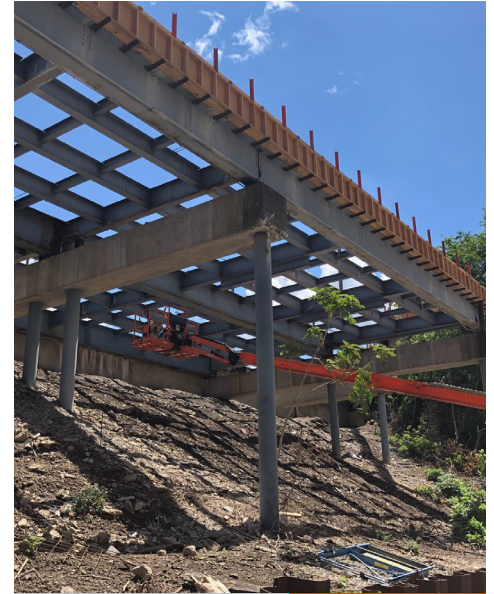
The ADM concrete bridge deck under construction
