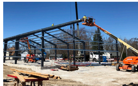
GEM erects steel at the Troy Township office/maintenance facility . RLI, design/build contractor, is self-performing site-work, concrete and masonry.
