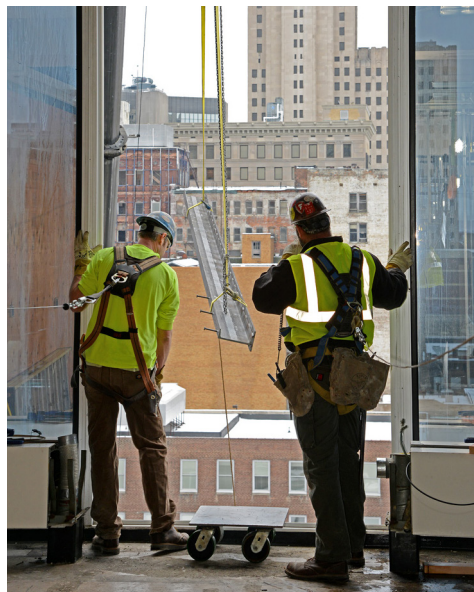
Hart, Inc. - Material for the private stairway connecting the 5th and 6th floors of the Hylant building was delivered and lifted through a window using a crane. Pictured are Jon Marshall and Matt Gurtzweiler .
