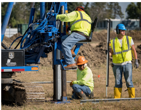
Above, L-R: Johnny Deleon and Frank Bernal of RLI, and Brad Plaucher of GEM drive piles for the ONU solar array. Below: Brian Cummings signs a commemorative solar panel presented to ONU.
