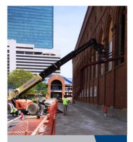
**GEM ironworkers** rig a large stair stringer to the second floor for the monumental stairway at the ProMedica Steam Plant building. The only way to place the stringers for erection was through a window.
