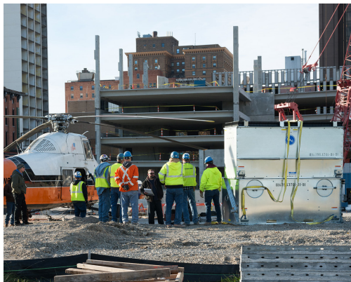
GEM placing the new rooftop cooling tower at the Toledo Renaissance Downtown Hotel.
