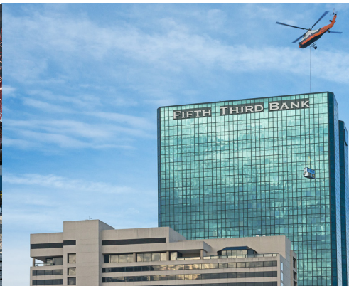
GEM placing the new rooftop cooling tower at the Toledo Renaissance Downtown Hotel.
