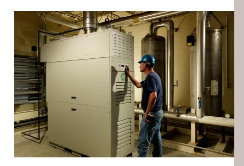
Combined heat and power systems generate on-site electricity to reduce the amount needed from a local utility.
