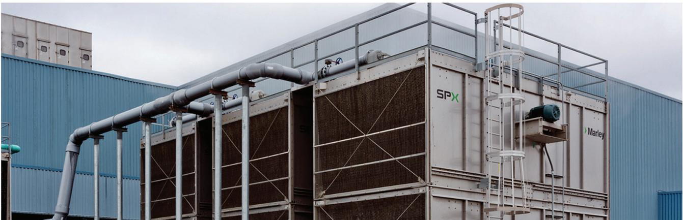
At Whirlpool Corp.’s Findlay, Ohio, dishwasher-manufacturing plant, company officials decided to add higher-efficiency cooling towers and pumps to help the plant increase control of utilities during high- and low-usage days.
