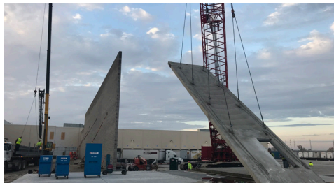
Tilt-up in progress at Walgreens' 395,000-square-foot expansion.
